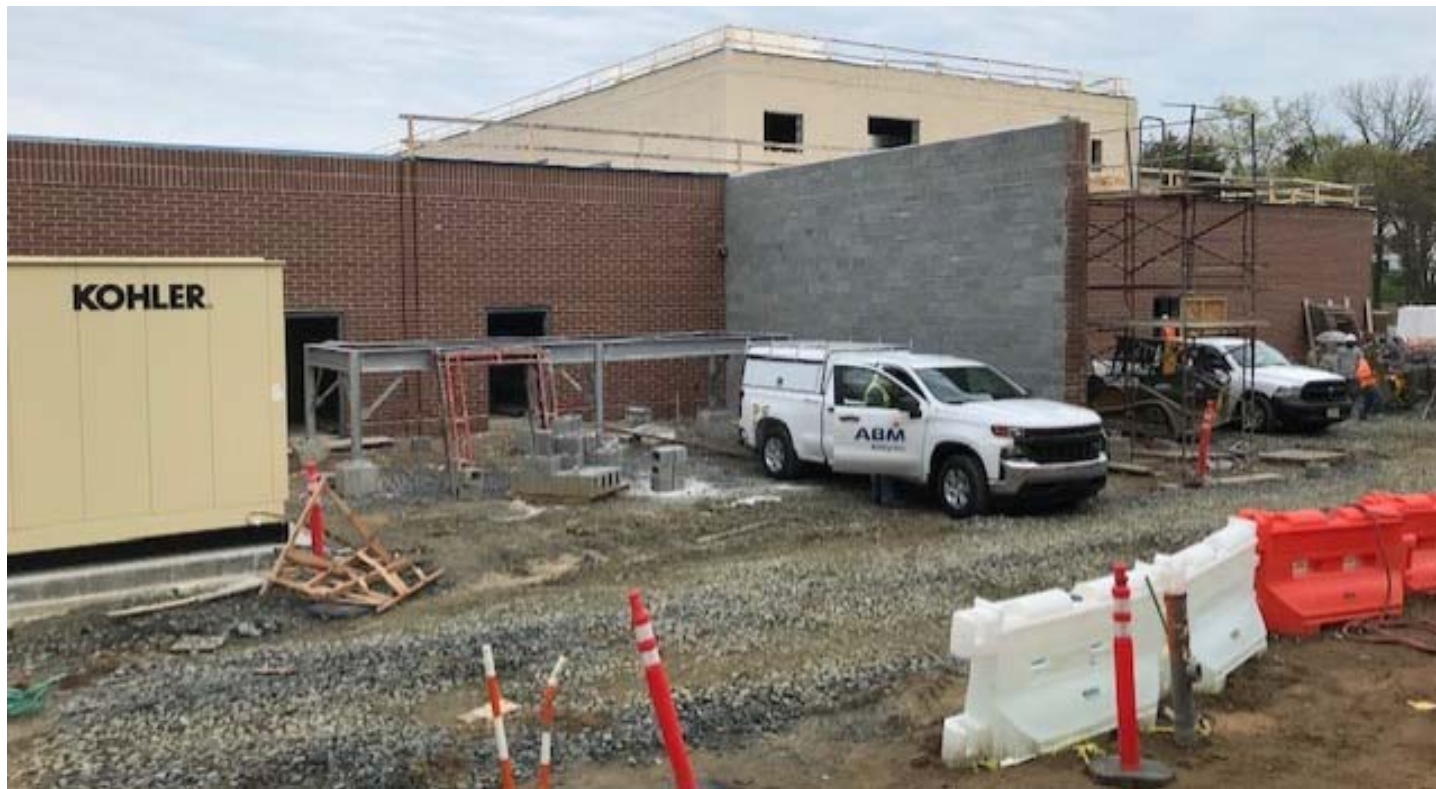
Mechanical yard, steel for cooling tower, generator, and screen wall
