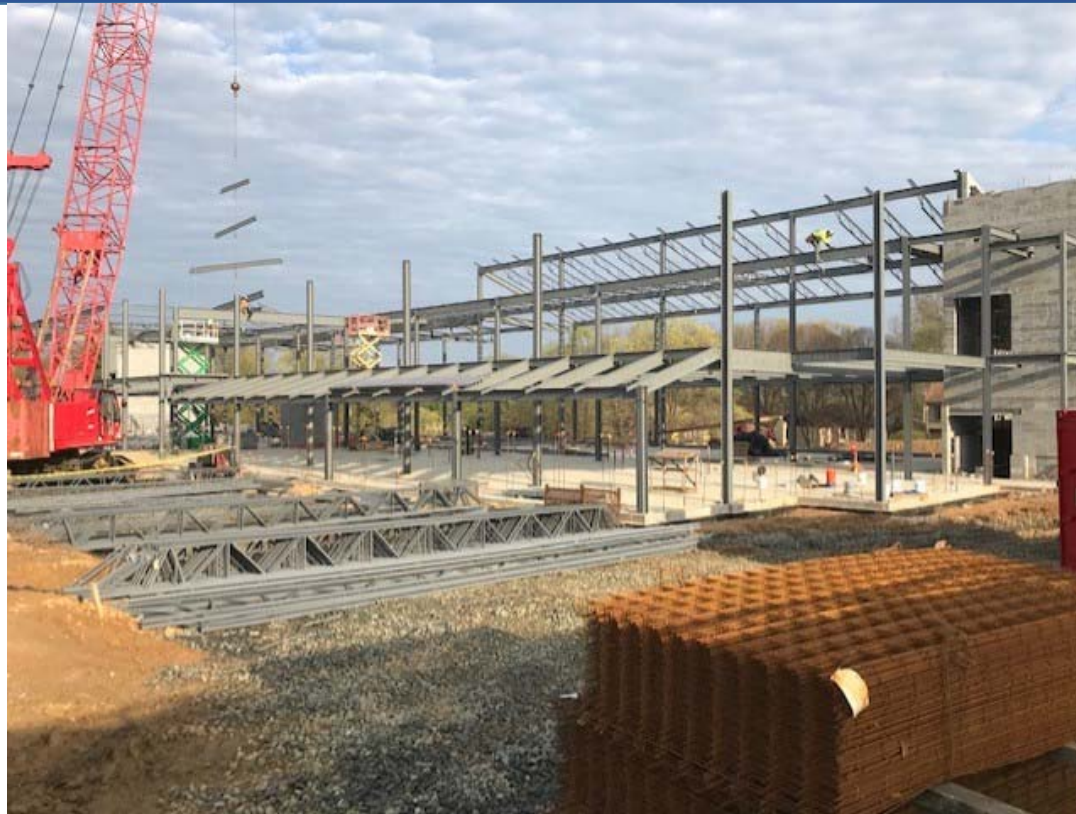
Structural steel at the two-story classroom wing
