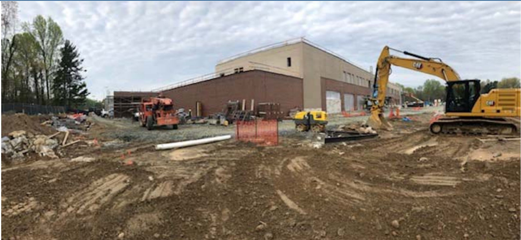
Panorama of service drive entrance at new kitchen
