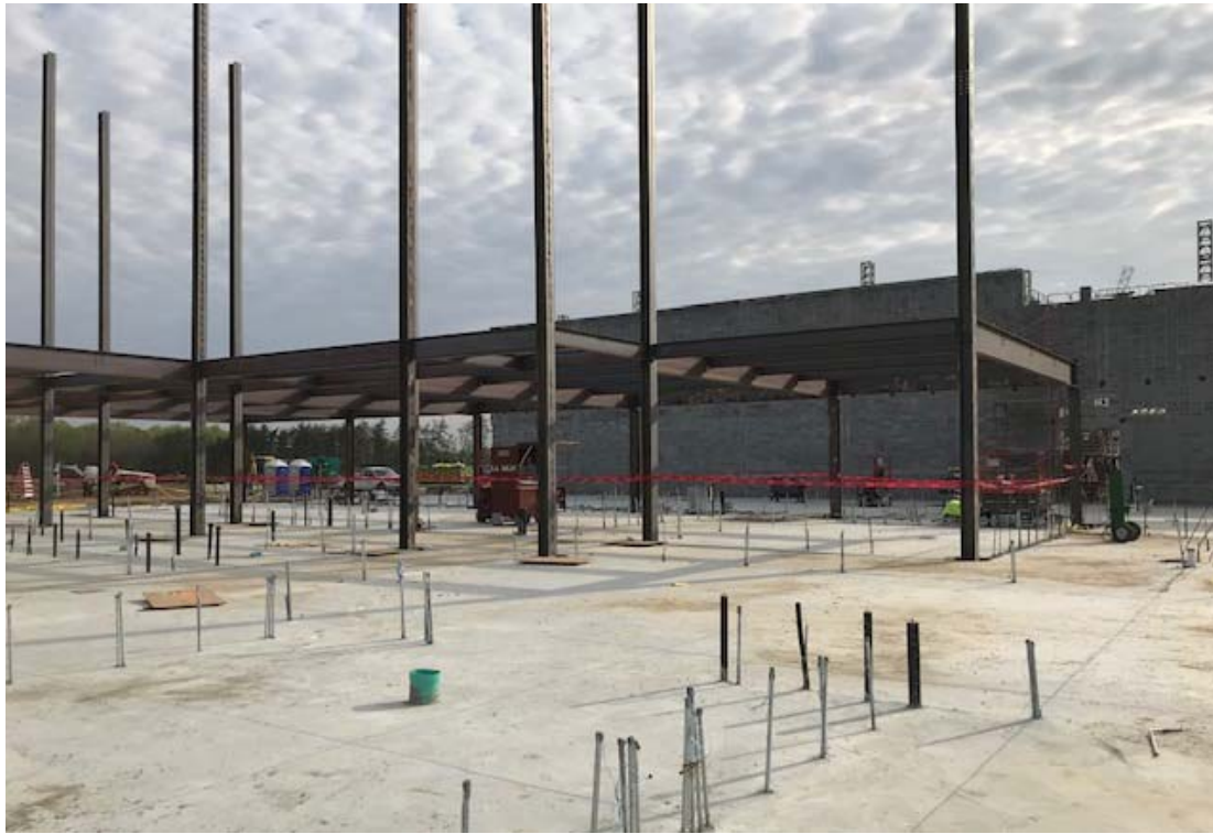
View from two-story toward the gymnasium
