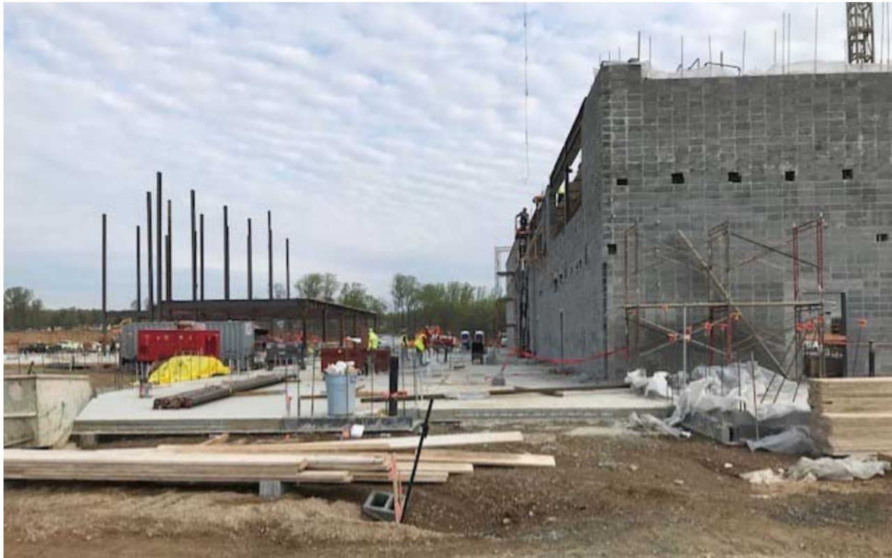
Photo of steel construction, slab and utility work, and masonry walls
