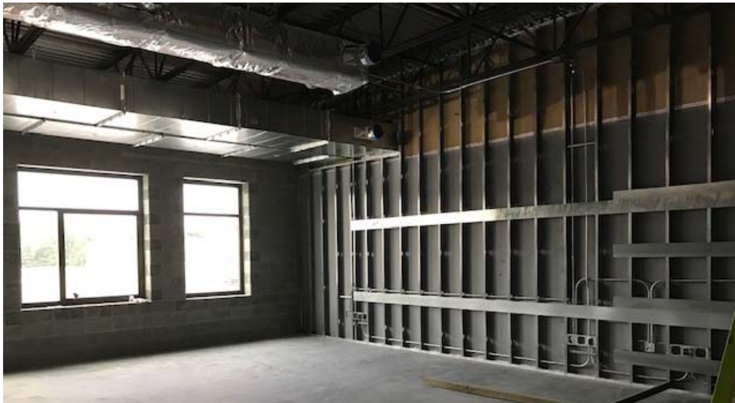
Typical classroom on second floor of Phase I
