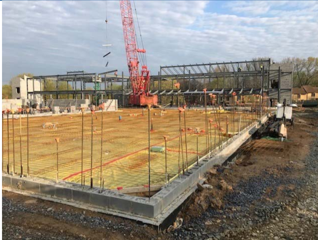
Foundation walls and concrete slab prep at the admin area
