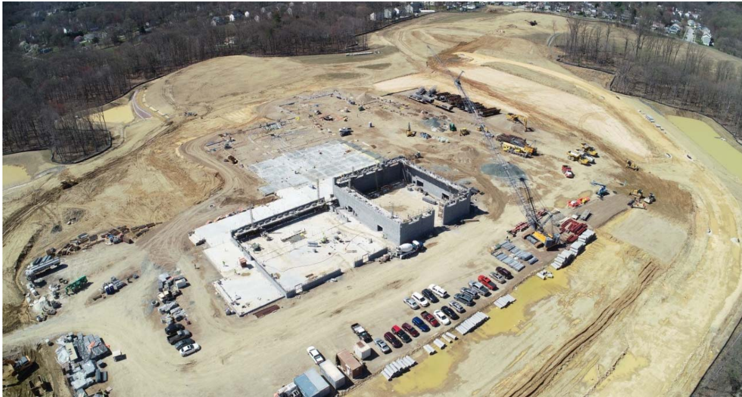
Aerial of construction site
