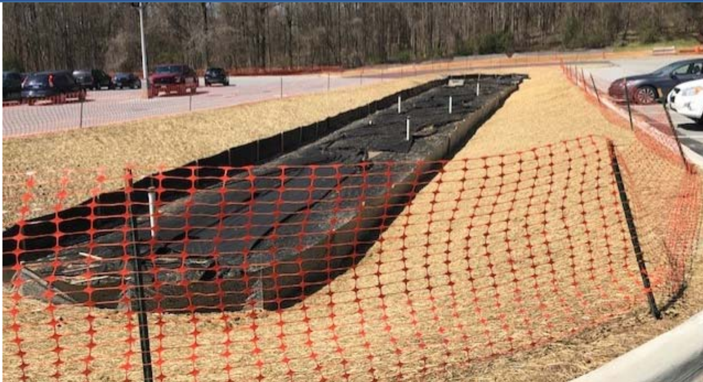
Storm water management facility at parking lot
