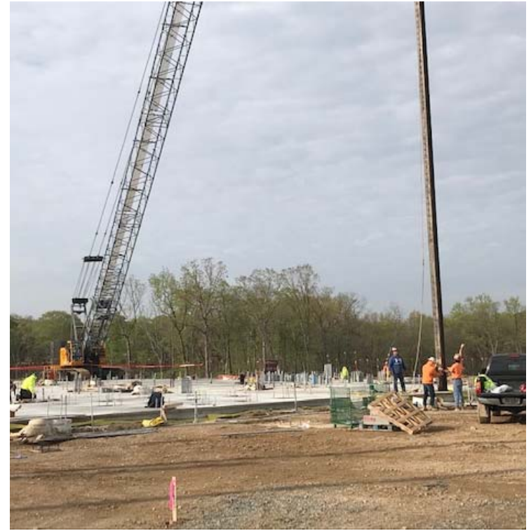
Setting a column
