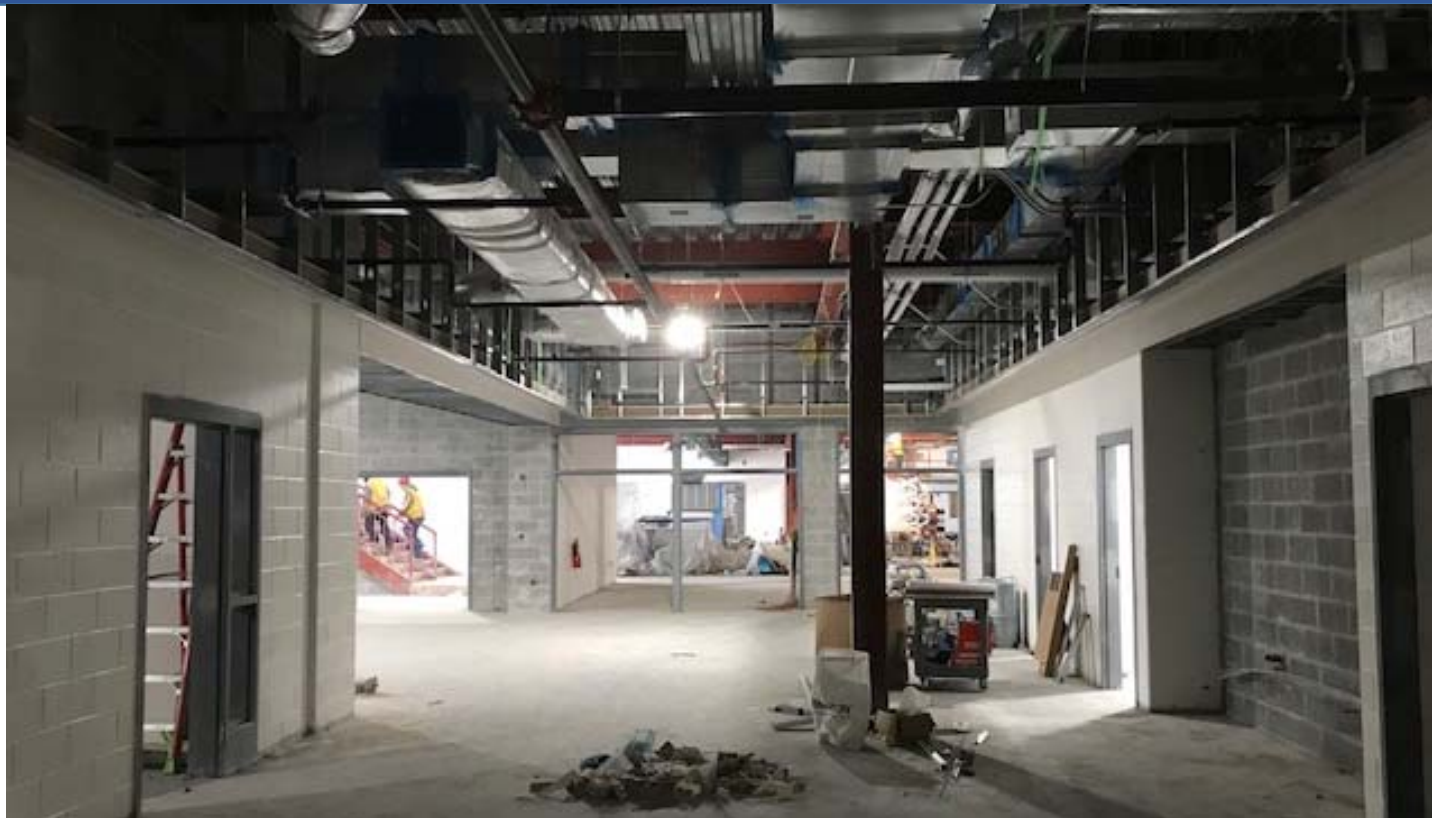
Photo of corridor and commons area at the cafeteria
