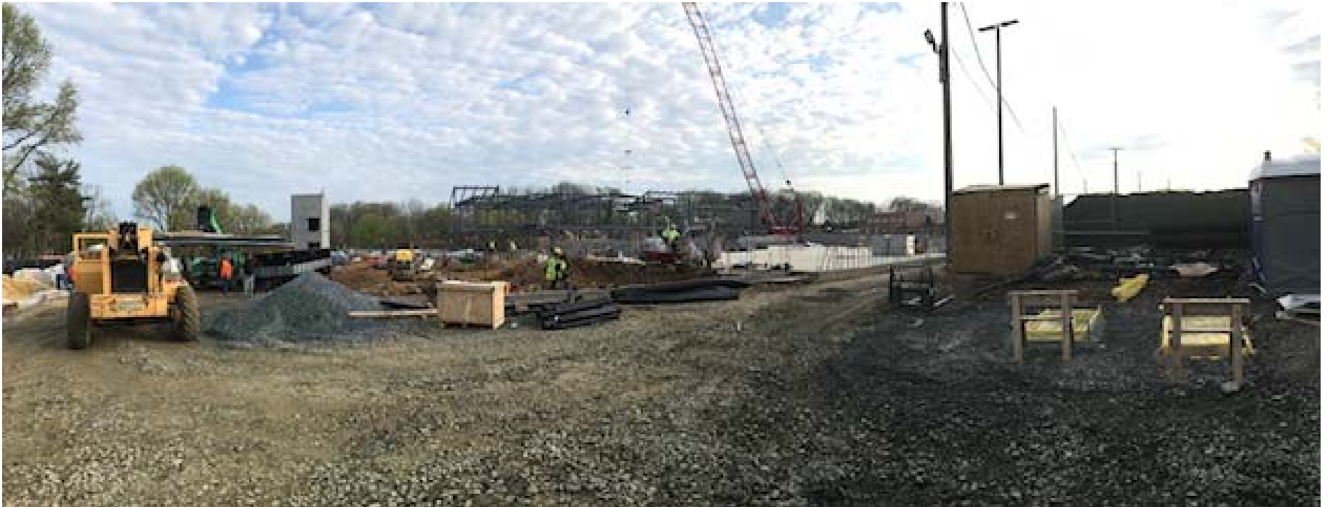
Panorama of the construction site with new facility centered
