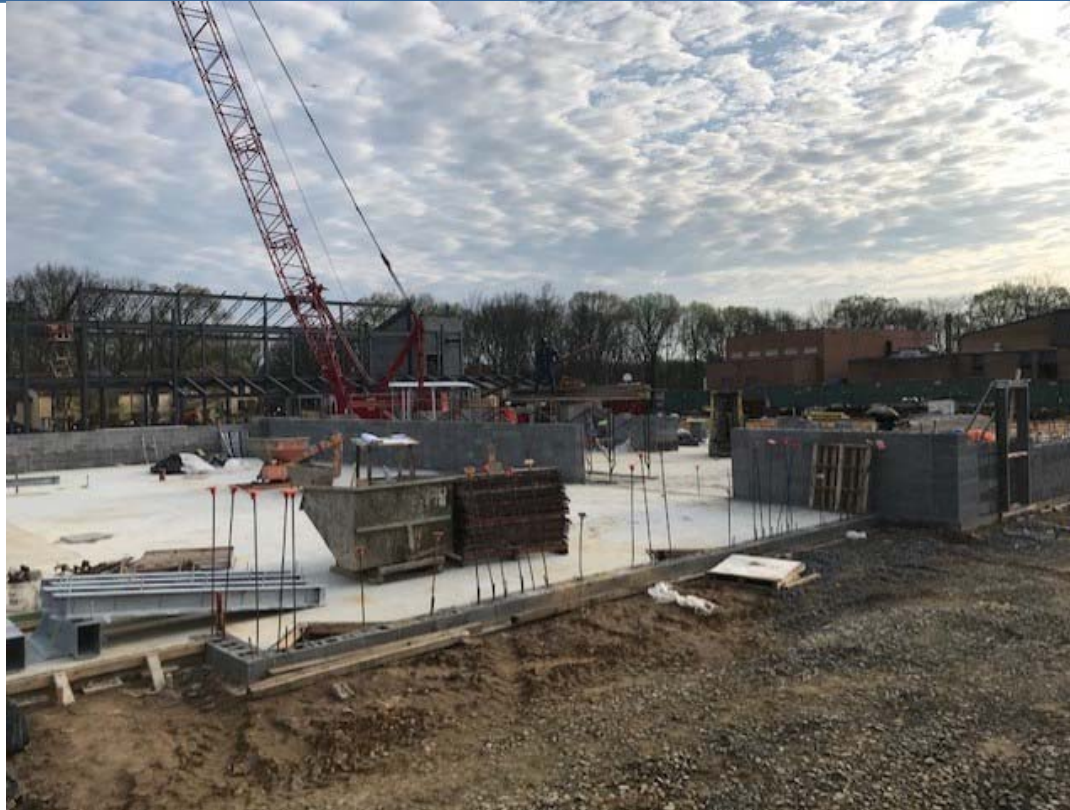
Slab on grade and masonry wall construction at the Gymnasium
